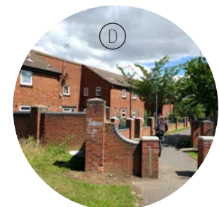
Radburn layouts on the Retford Road Estate aka Stepnall Heights/ Boughton Estate
